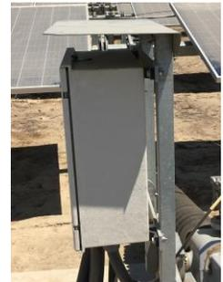
**Intra-field Communication:** Master/Slave communication is done via a RS485 wired network, or wireless. A wired network can comfortably span 1km, is known for high reliability, but may also require more installation effort. The wireless interface operates at 916MHz. The sparsity of block trackers can make wireless networks a challenge to operate, even with directional slave antennas.
