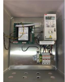
If the existing control enclosures are in good condition, and of sufficient size, a simple backplane swap can be made, thereby minimizing conduit rerouting and power cables. If a new enclosure is warranted, a fiberglass model is warranted to facilitate ease of installation.
